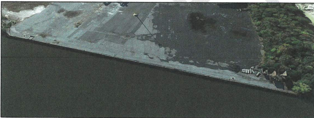
Figure 1.2: Steel Bulkhead 31B
